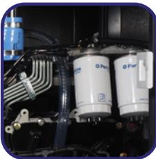
Fuel particle separator filter
